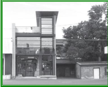
Example of Inappropriate Renovation
