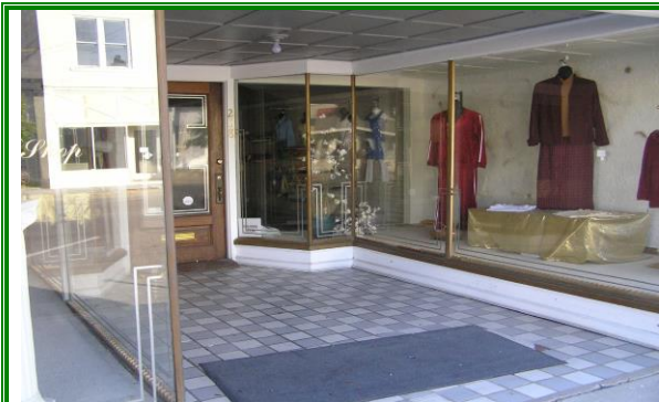
Appropriate Storefront Preservation
