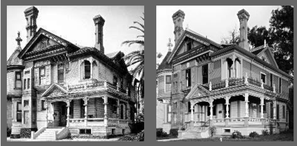
Preservation of the exterior of the Hale House, Los Angeles, California, involved repainting the exterior walls and decorative features in historically appropriate colors. An excellent example of the Preservation treatment focused upon the ongoing maintenance of historic materials and features. Photo: Before, NPS files; After: Bruce Boehner.
