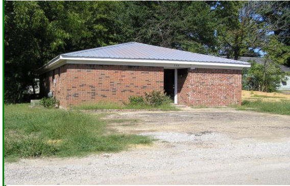
Incompatible new construction
